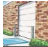
A dock lift is the loading dock at a ground level building.
