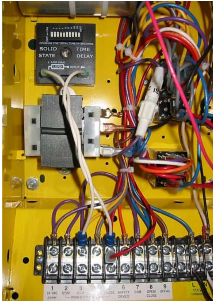
Photo #2 (Timer Mounting in Operator)
