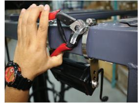
7. Place plastic clamp end piece over sharp end of clamp strap so there are no sharp edges.
