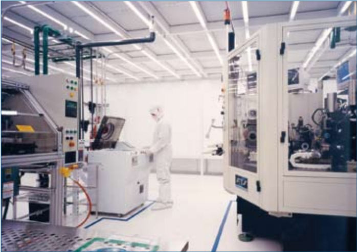
Elevated wall panels for low wall returns in circuit board manufacturing facility.
