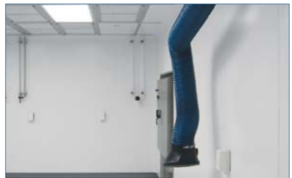
The double wall design of PharmaWall allows equipment, ductwork and mechanical to be installed within the wall cavity
