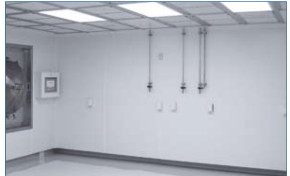
Raised air walls eliminate the need for a grill and provide a more cleanable detail, reducing crevices in the room.
