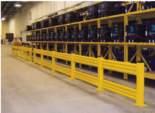
Guarding battery racks
