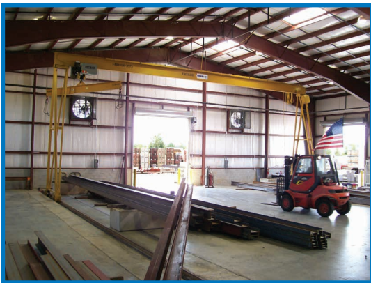
A 7.5-ton Motorized Spanco PF Gantry Crane used to move truckloads of long steel beams at a building material supply center
