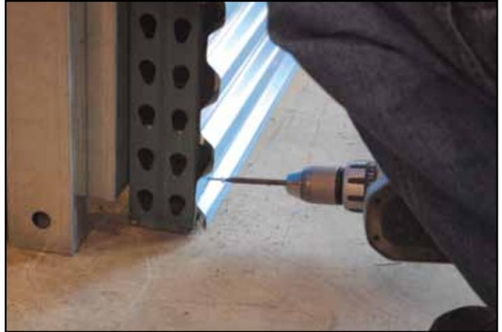
**19.5** If side panels are used to separate a secure rack from an unsecure rack, fasten the panels with tek screws to the interior of the secure rack. Use a tin snips to create notches for the rack's horizontal supports. Use 6 screws per panel.
