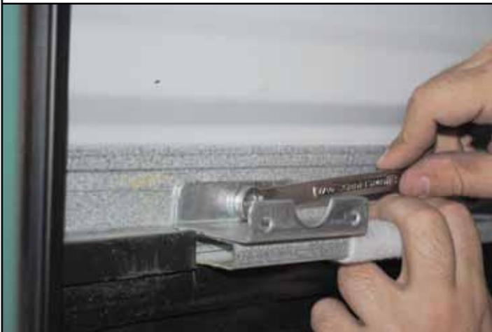
**12.** Attach door keepers to each end of the door's bottom bar using the 1/4" - 20 carriage bolts.
