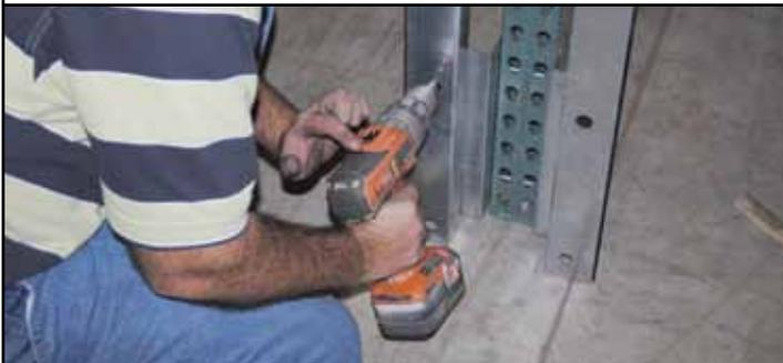
**24.** If multiple bays are to be enclosed with the Rack-Lock system, install neighboring rack mounts, door and guides. Center jambs may then be installed between the guides of the adjacent racks. Fasten with tek screws through the prepunched holes within the guides.
