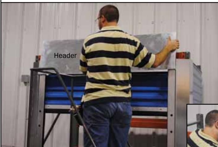
**25.** Headers may be installed after jambs are installed on both sides of a door opening. Slide the header into the gap between the guides and jambs. Secure it with tek screws from both above and below the header. Install tek screws in the remaining guide holes to fasten the guide to the jamb.
