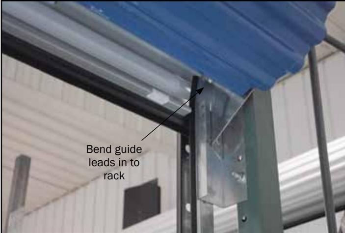
**10.** Holding the door securely so that it does not unwind, cut the bands and feed the door into the guides. The top edges of the guides should be bent into the rack to allow for smooth operation.
