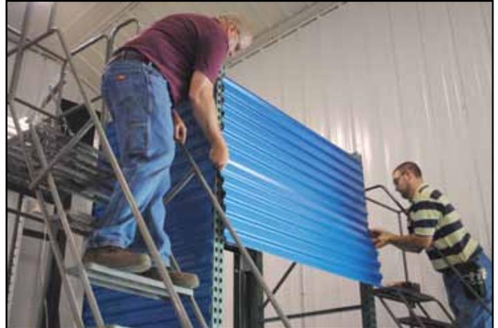
**27.** Position and fasten the rear corner trims (included with the optional side and back of rack closure system). Tek screws may be used as a temporary fastener. For a permanent and more secure attachment, install security bolts as was done during corner jamb installation.
