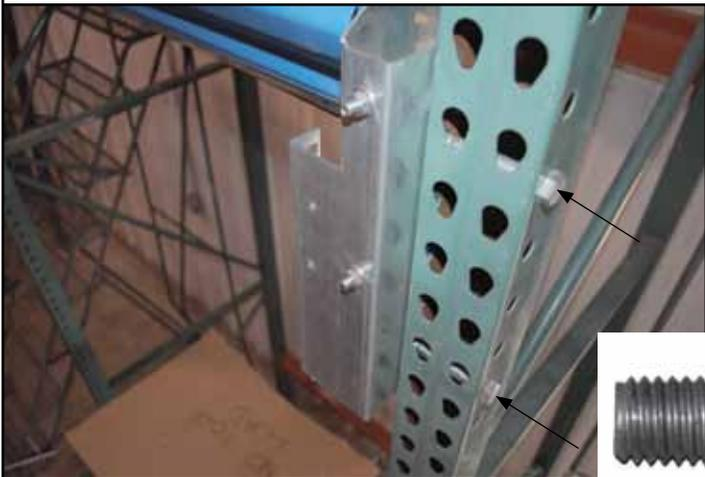
**5.** Align the holes on the upper mounts with a set of holes in the rack and loosely secure with 4" hex bolts and nuts. These bolts will be tightened further in step #14.
