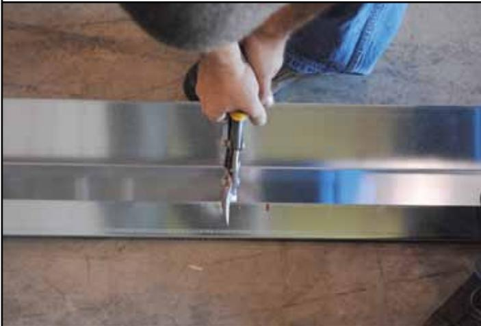
**18.** Cut the upper and lower extents of the area, and fold the flap inward or cut it out entirely.
