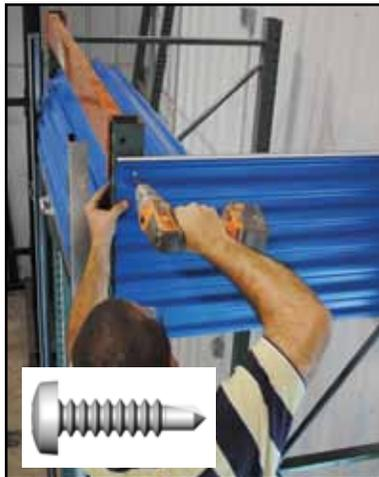
**19.** If Trac-Rite's optional side and back of rack closure system or other side closure material will be installed, add it at this time.
