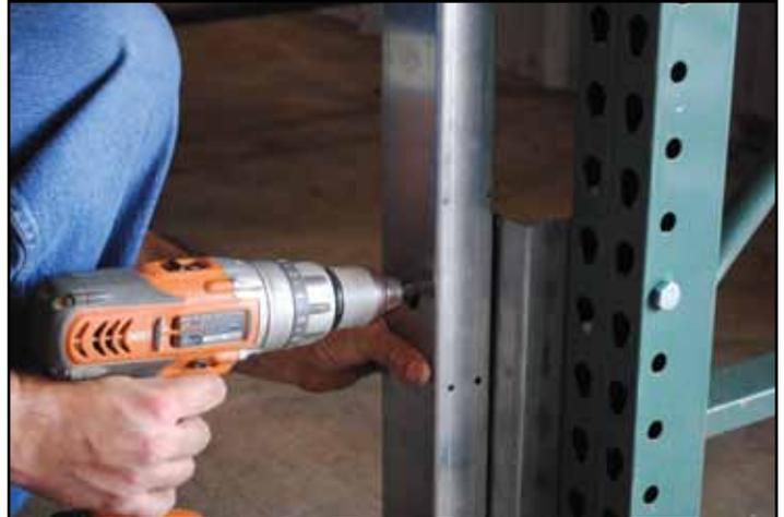
**15.** The latch side jamb must be notched to allow room for the latch to slide closed. Measure from the floor to the bottom of the latch opening.
