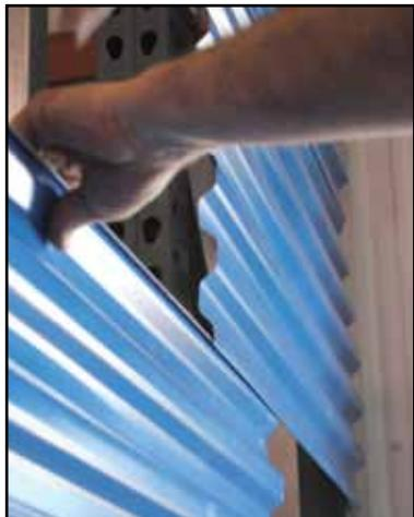
**19.3.** Hang the remaining panels using the "hooks" but do not fasten yet. Slide them in to place from the side. With all panels in place, the bottom edge should hang just above the floor.
