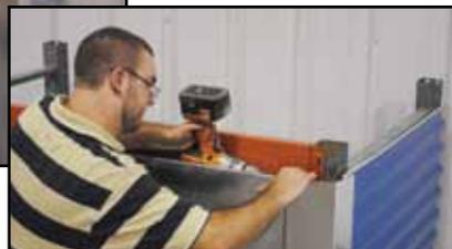
**26.** If Trac-Rite's side and back of rack closure system or other closure materials will be used, install now. If using Trac-Rite's rear panels, install them using the same procedure as the side panels.
