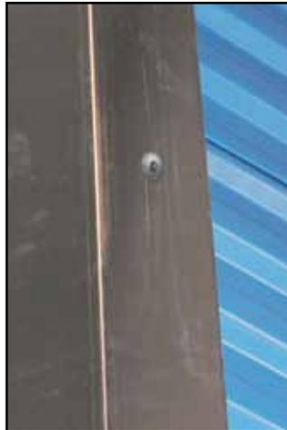
**22.** To install the corner jamb security bolts, 1/2" holes must be drilled. Select locations approximately 1-2' from the top and bottom of the rack, and insert the drill bit through the rack to drill through the corner jamb.
