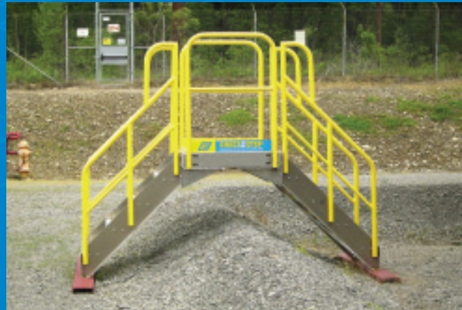
Four stair berm crossover.
