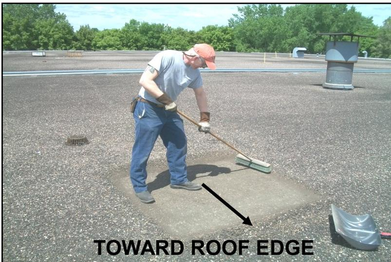
On gravel topped roofs, BUR, Ballasted etc... thoroughly sweep away all gravel, dirt and dust over the area where you will locate the anchor. Allow at least 3 feet of swept area in front of the Anchor (direction toward roof edge).
