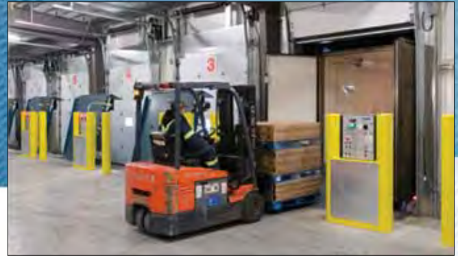
COLDSTORAGE™ vertical levelers in a distribution facility. Installation included custom control panel stanchions, bollards and TRUCK-LOCK® vehicle restraint systems.
