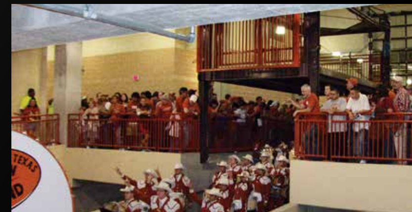
Stadium Concourse Lift – F Series Mechanical VRC 12' high clearance for the University of Texas Longhorns; 12,000 lbs. lifting capacity; fully ascends/descends in 30 seconds.
