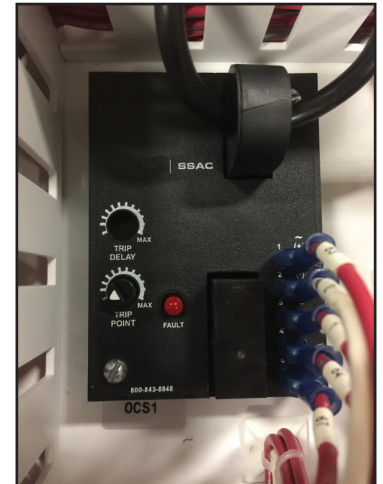
Overcurrent Sensor Figure 21-1
