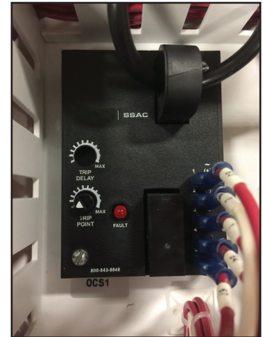
Overcurrent Sensor Figure 21-1
