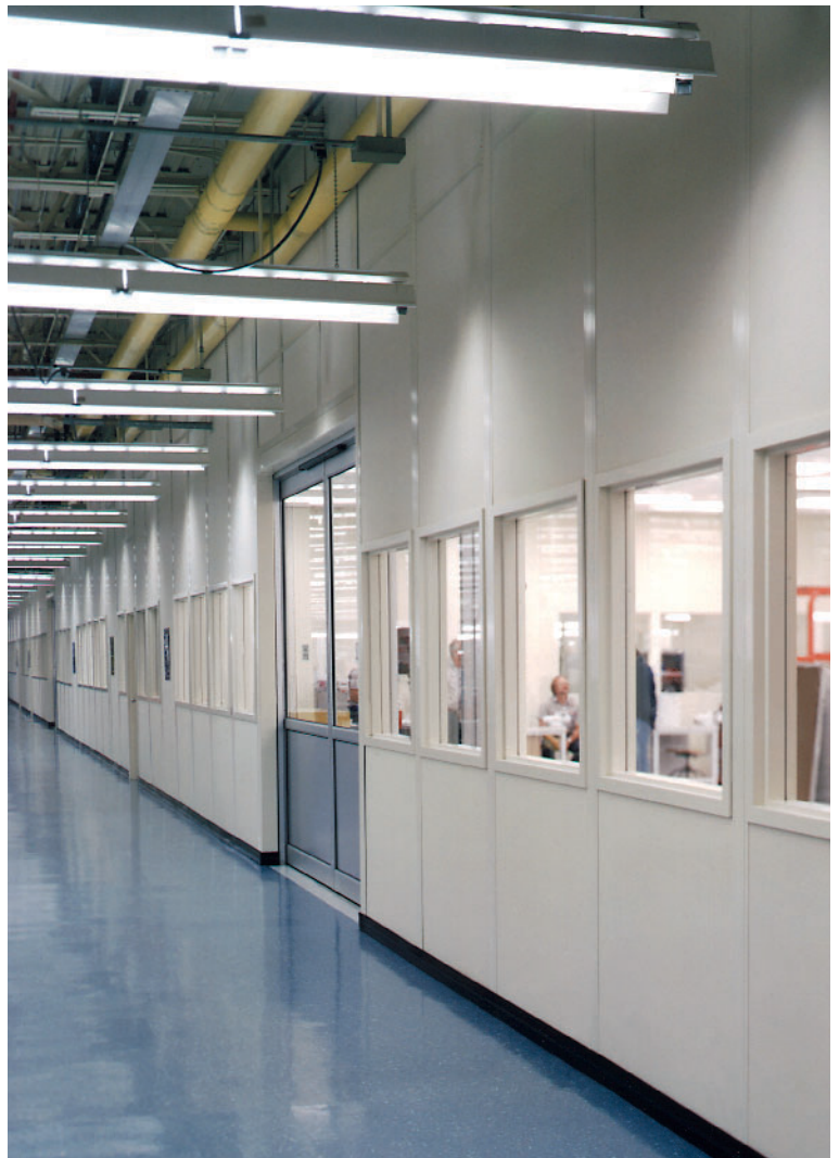
Environmentally-controlled enclosure for manufacture of intricate electronic components. Electronic sliding door.
