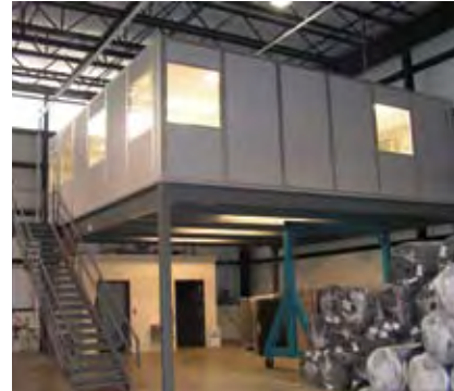
Elevating this shipping manager's office maintains work space below while creating a quieter working environment.
