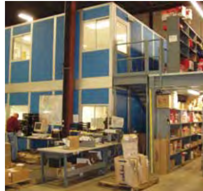
A modular two story serves as office space and a quality control lab while the adjacent mezzanine creates two levels for materials storage.
