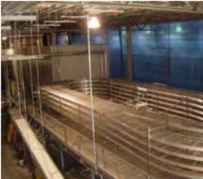
This bakery conveyor platform enables this national bakery chain to move an automated process overhead.
