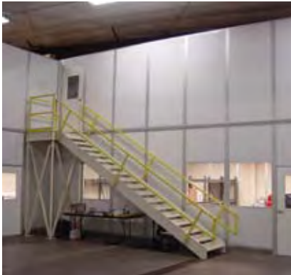
This integrated system includes inventory storage on the lower level and a secured storage platform upstairs.
