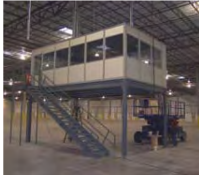
This plant manager's office was built on top of this mezzanine to aid in supervision of plant personnel and equipment.
