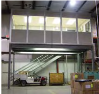
This modular system was integrated with our mezzanine to create a new office space while keeping the floor below open.
