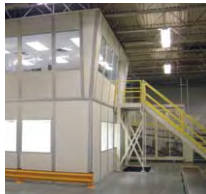
The walls on the top floor of this control room are angled out to provide plant personnel with a better view of the production line below.
