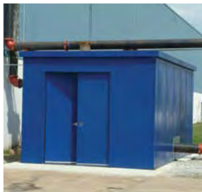
20'x12' Durasteel pump house with solid wall construction that includes a double door for equipment maintenance.
