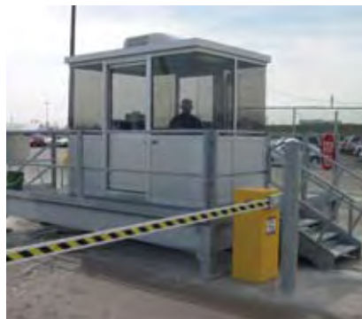
An elevated platform for this access control booth raises the operator height consistent with truck driver height for easier transactions.
