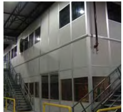
This modular two story was placed in an unused part of this plant to create needed office space without the substantial cost of new construction.
