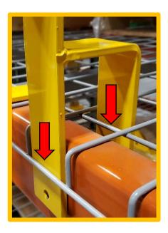
(2) Slide bolt (Grade 8) through the holes on the legs of the Beam Pallet Stop. Secure the bolt in place with the nylon hex nut. Tighten nut until Beam Pallet Stop is snug and securely in place.
