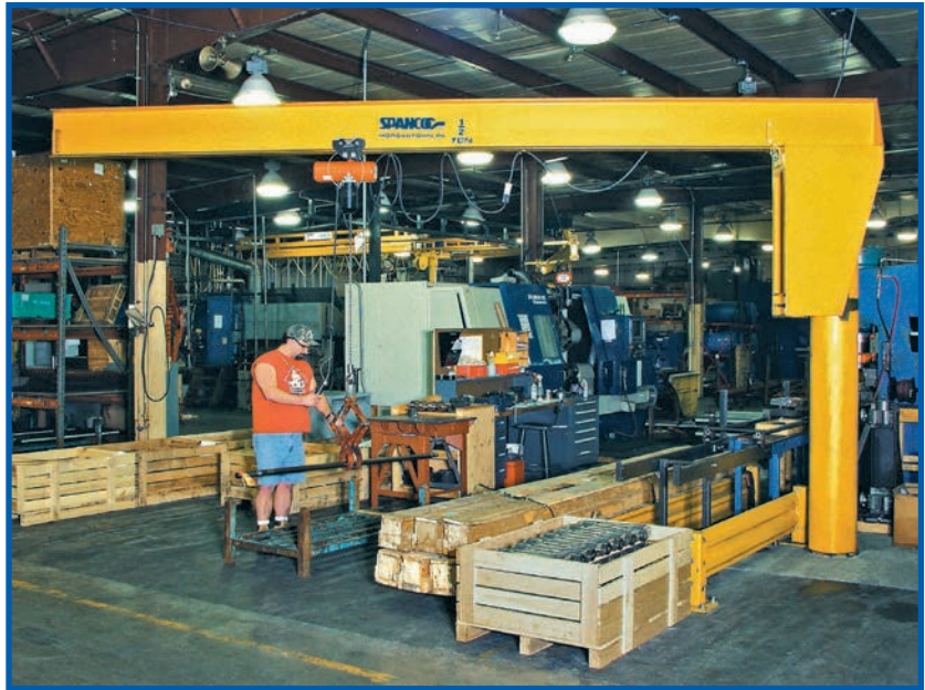
A Spanco 102 Series Freestanding Jib Crane lifting solid metal bars weighing up to 1/2 ton.
