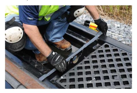
16.) If using grates as a walking surface for the Ultra-Track Pans, Composite Model, positon five grates in each Side Pan, using the grating locator positions on the pans.
