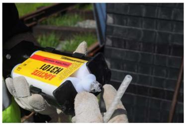
Using the adhesive dispenser, apply adhesive to each side of the endwall of each pan.
