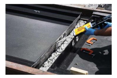
Push the second pan into the first pan, while keeping the first pan in place, carefully aligning the flow-through holes in each endwall. Once the two pans are together, use C-Clamps to tighten the two pans together between the two flow through holes and on the outside of each flow through hole.
