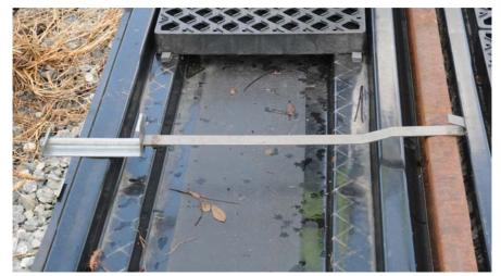
NOTE: Side Pan Rail Clip shown ON TOP of Track Pan for illustration purposes only. Actual installation will be underneath the Track Pan and rail.
