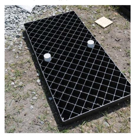
10.) Positon ten grates in each Center Pan, using the grating locator positions on the pans.
