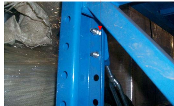
X-brace mounting bracket hardware (M12 bolts, nuts, lock washers & washers)
