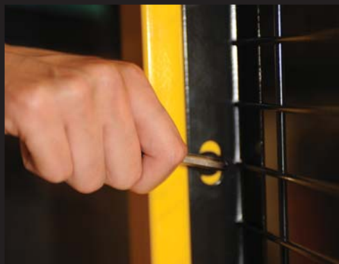
OSHA-COMPLIANT TOOL REMOVABLE BOLTS ARE ACCESSIBLE FROM INSIDE THE ENCLOSURE
