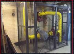
Secure & limit access to electrical panels; backflow, mechanical & elevator equipment; meters & pipes.
