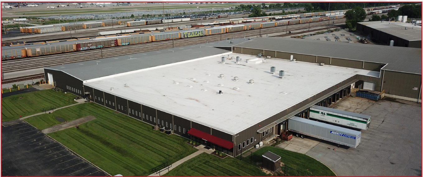
Aerial view of the WireCrafters facility.
